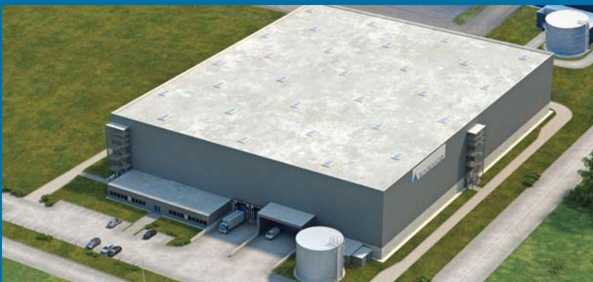
The Perspective of upcoming Iron Mountain Archive Centre at Gazeley's Magna Park Rhein-Main in Germany
