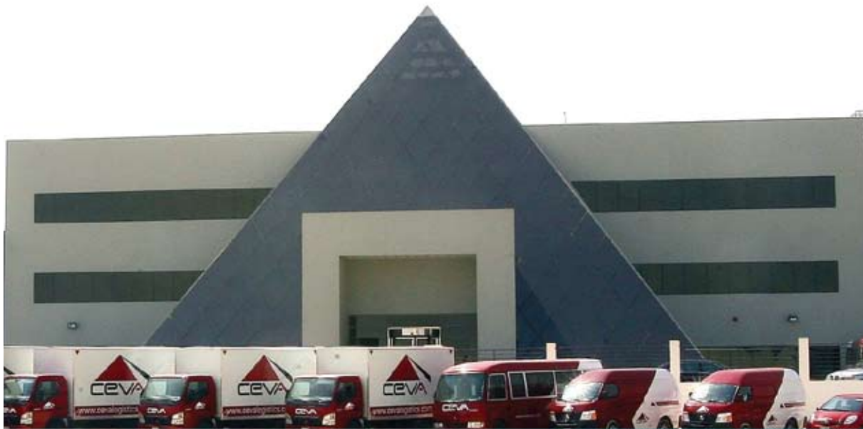
CEVA Logistics' new regional headquarters in Jafza
