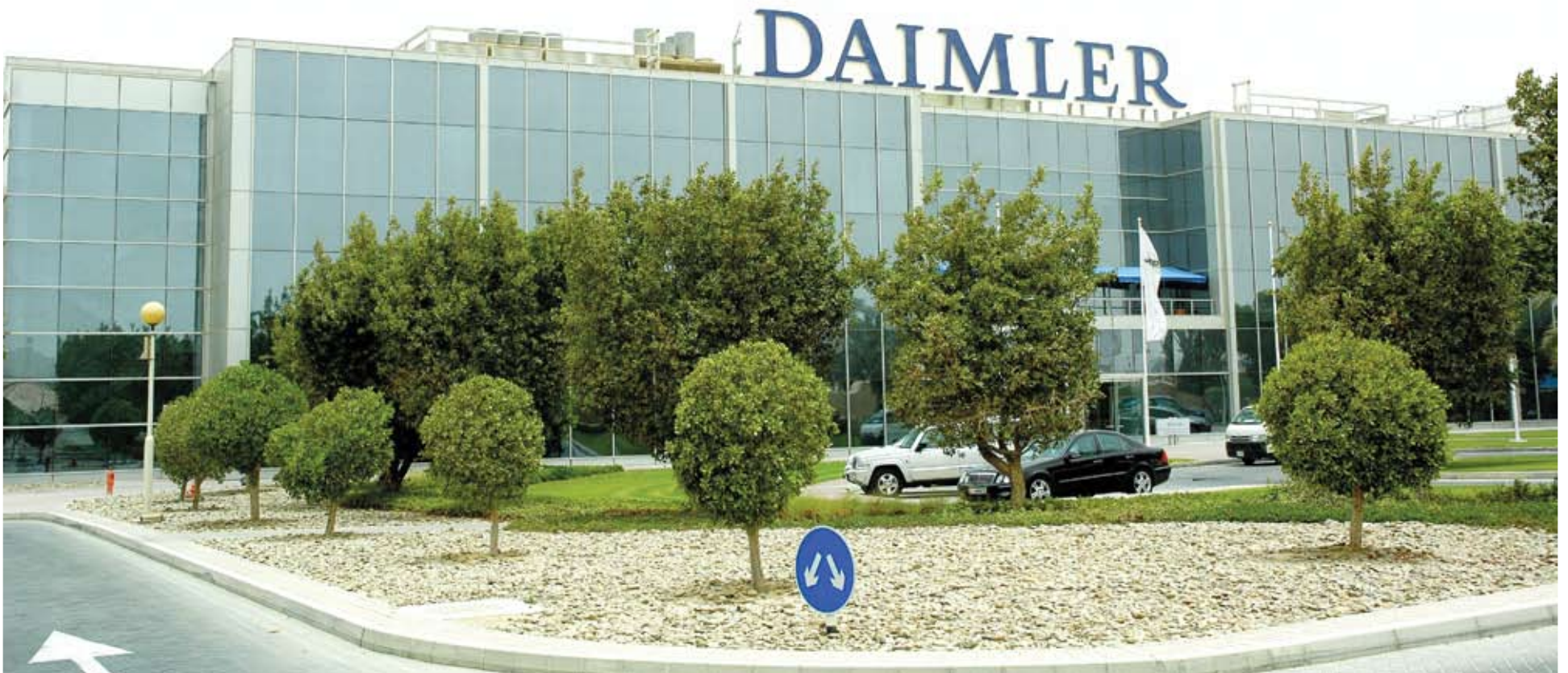
Daimler Regional Headquarters Building in Jafza
