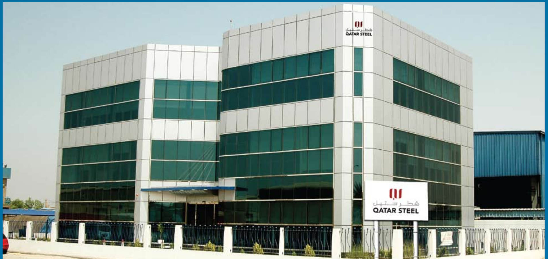
Qatar Steel Company FZE in Jebel Ali Free Zone
